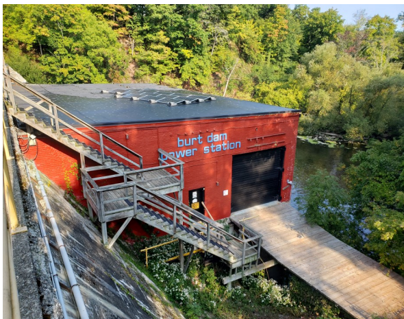
Below: Burt Dam power station September 2020
