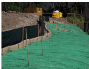
Silt fence with erosion control blanket
