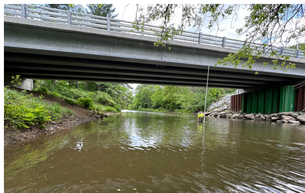
Resilient NY studies evaluate how infrastructure interacts with waterways, as shown here at a Genesee River bridge.
