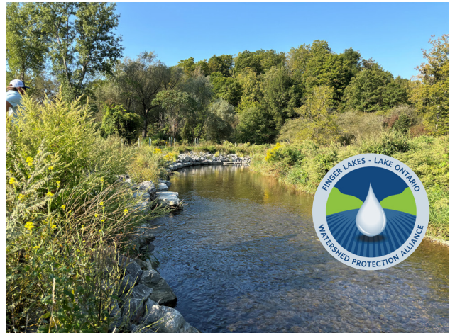
Streambank stabilization and restoration along Wiscoy Creek in the Upper Genesee River
