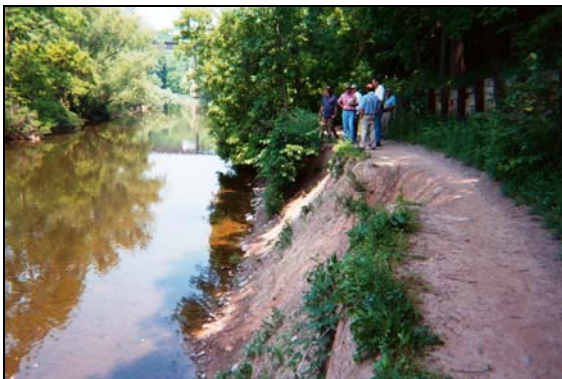
Excessively eroded streambank and trail below Burt Dam in 2002 and streambank after Phase I restoration
