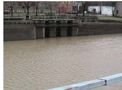
Figure 5-3 Hydraulic Connection between the Erie Canal and Eighteenmile Creek
