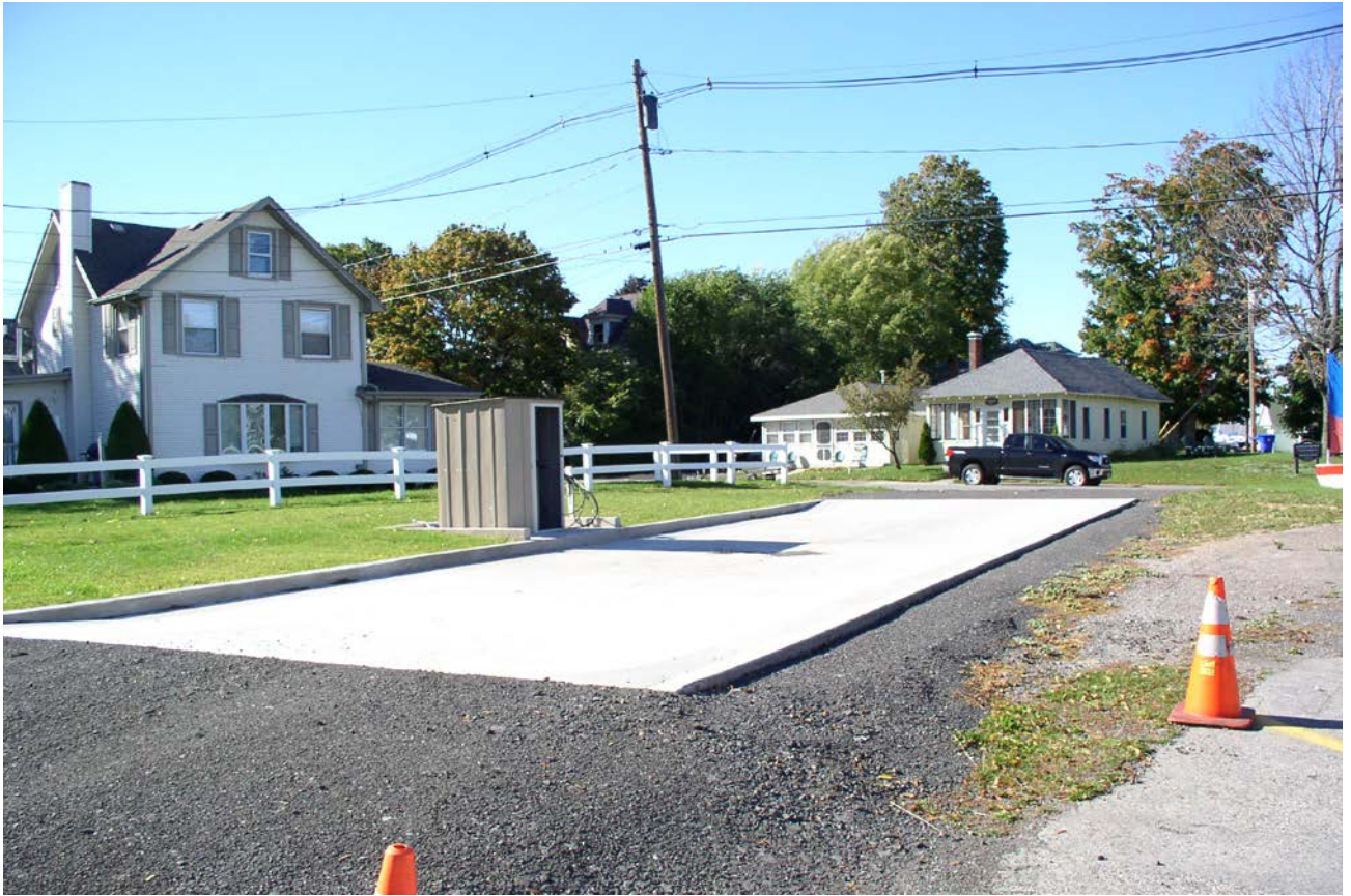
COMPLETED INVASIVE SPECIES BOAT WASH PAD AT OLCOTT HARBOR
