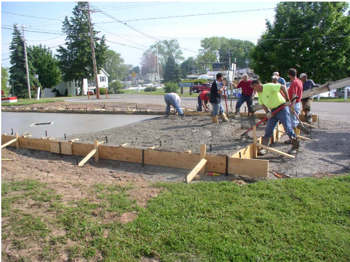
CONSTRUCTION OF INVASIVE SPECIES BOAT WASH PAD AT OLCOTT HARBOR
