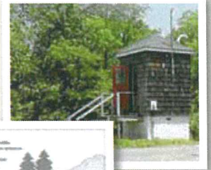
Gauge Station (House) www.geology.com
